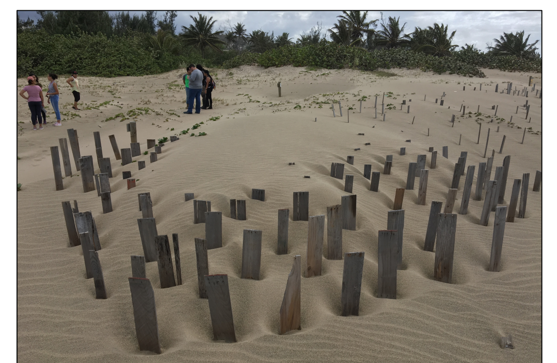
Figure 10. Accumulation of sand by a biomimicry matrix easternmost dune restoration site in Finca Nolla Camuy, PR.
