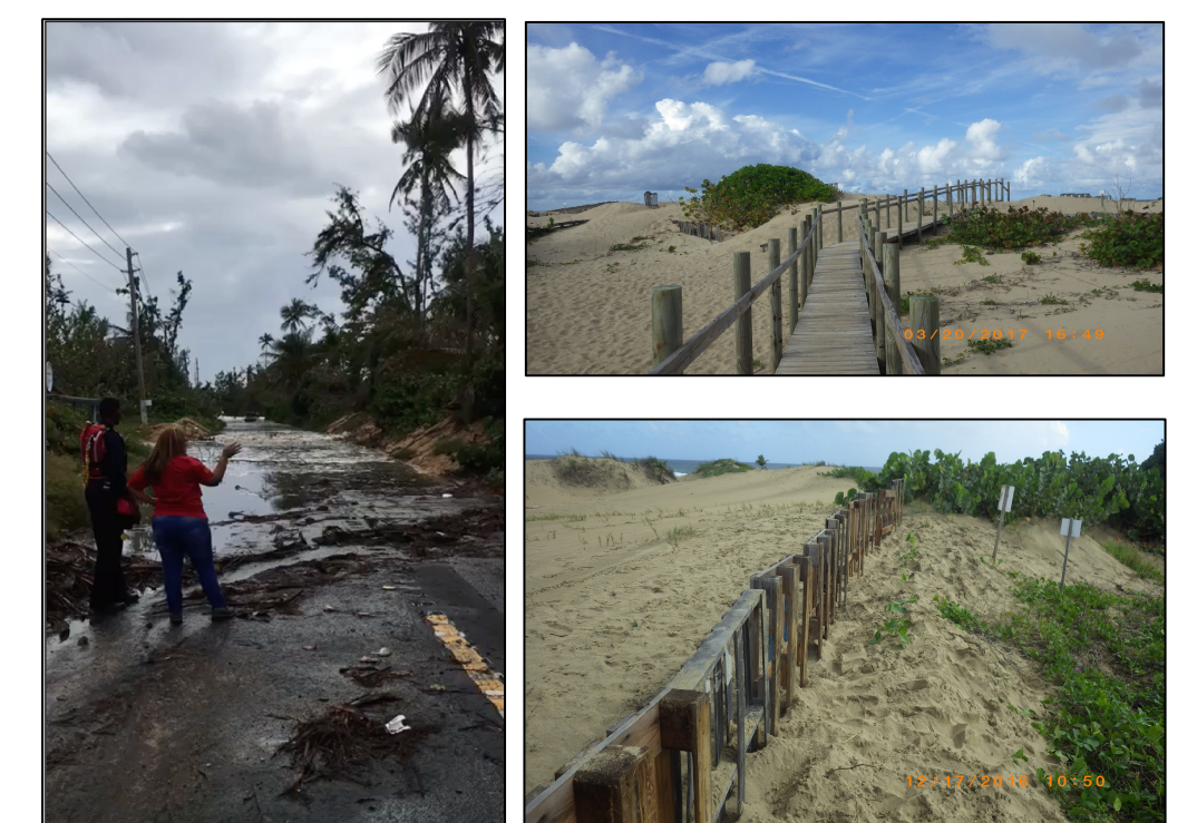
Figure 6. Flooding of road PR-187 in Loiza. Water entered the roadway through breaks in the dune caused by heavy foot traffic (left). These breaks can be reduced by re-directing foot traffic away from these areas by installing wooden boardwalks in sensitive areas of the dunes (right).
